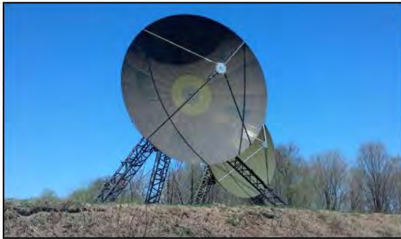
Figure 5. Building 1600 28-Foot Antenna (Typical)
